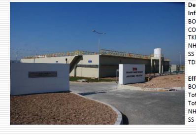
Design Requirements Influent average loadings: BOD 1,200 mg/l 2,000 mg/l COD. TKN 61 mg/l  $NH_3 - N$ 55 mg/l SS 450 mg/l 5,000 mg/l TDS Effluent standards BOD 30 mg/l Total N 15 mg/l Total P 1 mg/l 1 mg/l  $NH_3 - N$
