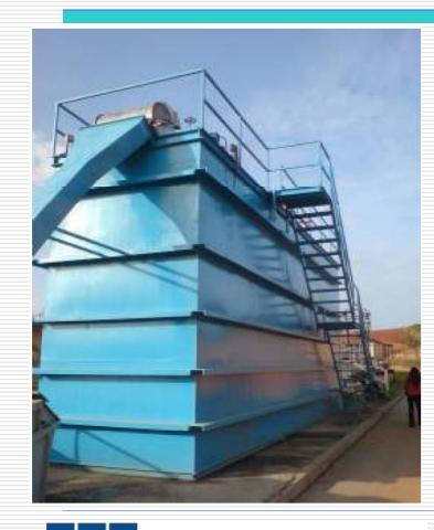
**Design Requirements** Influent Average Loadings: BOD 300 mg/l COD 600 mg/l TKN 45 mg/l NH<sub>3</sub> – N 40 mg/l SS 300 mg/l TDS 5,000 mg/l
